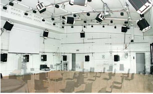
Figure 6: The IEM-CUBE is a 24 channel hemispherical Ambisonics system.
